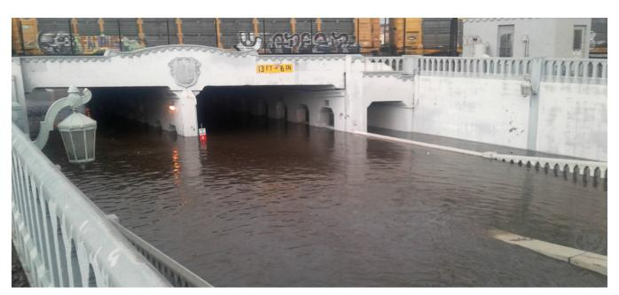
Limited stormwater infrastructure relies on Tucson's roadways for water conveyance during rain events. In addition to impeding travel during major storms, this also leads to increased pavement maintennace needs.
