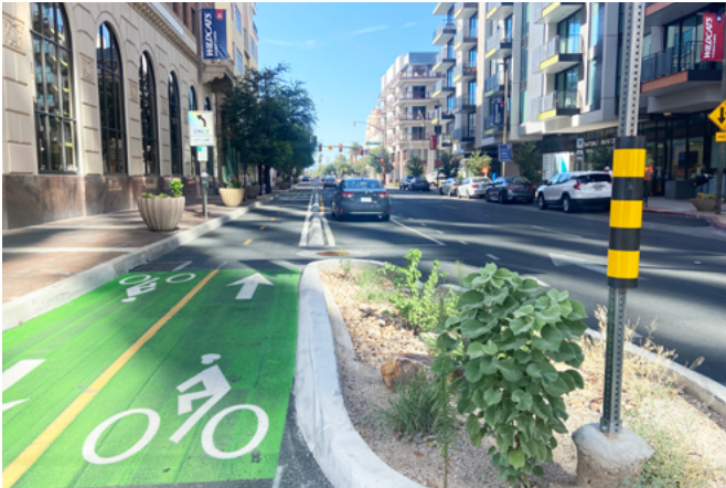
Stone Ave Bike Boulevard - GSI bike lane buffer
