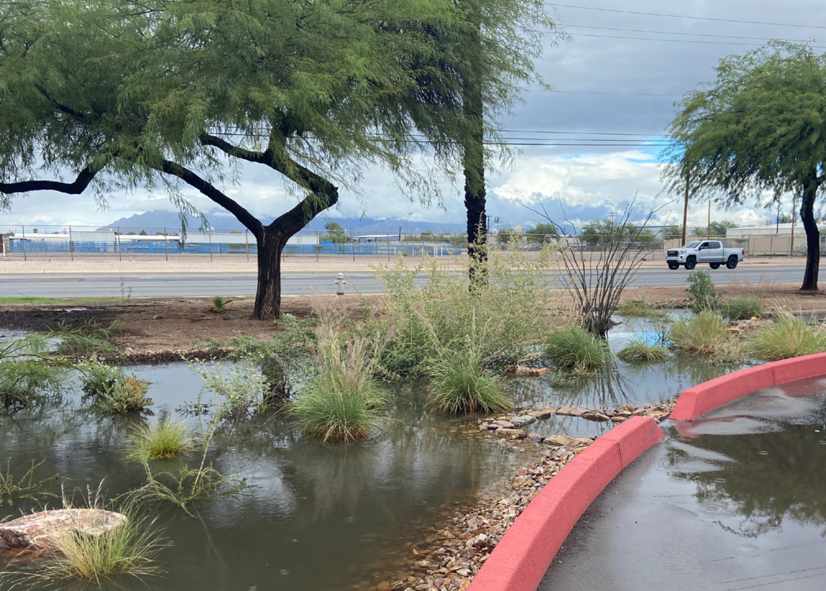
Above: Rudy Garcia Park Parking Lot GSI Basins Cover (left to right): Pantano ROW Project , GSI Maintenance at Lower Lincoln Park, Rudy Garcia Park GSI Median
