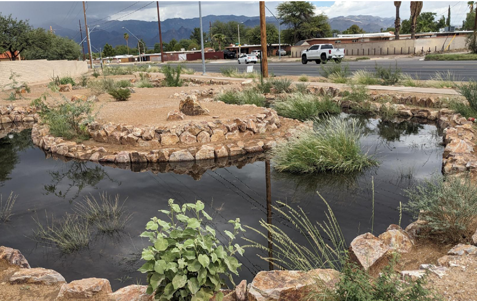
Newly constructed Pantano right-of-way project after a rain
