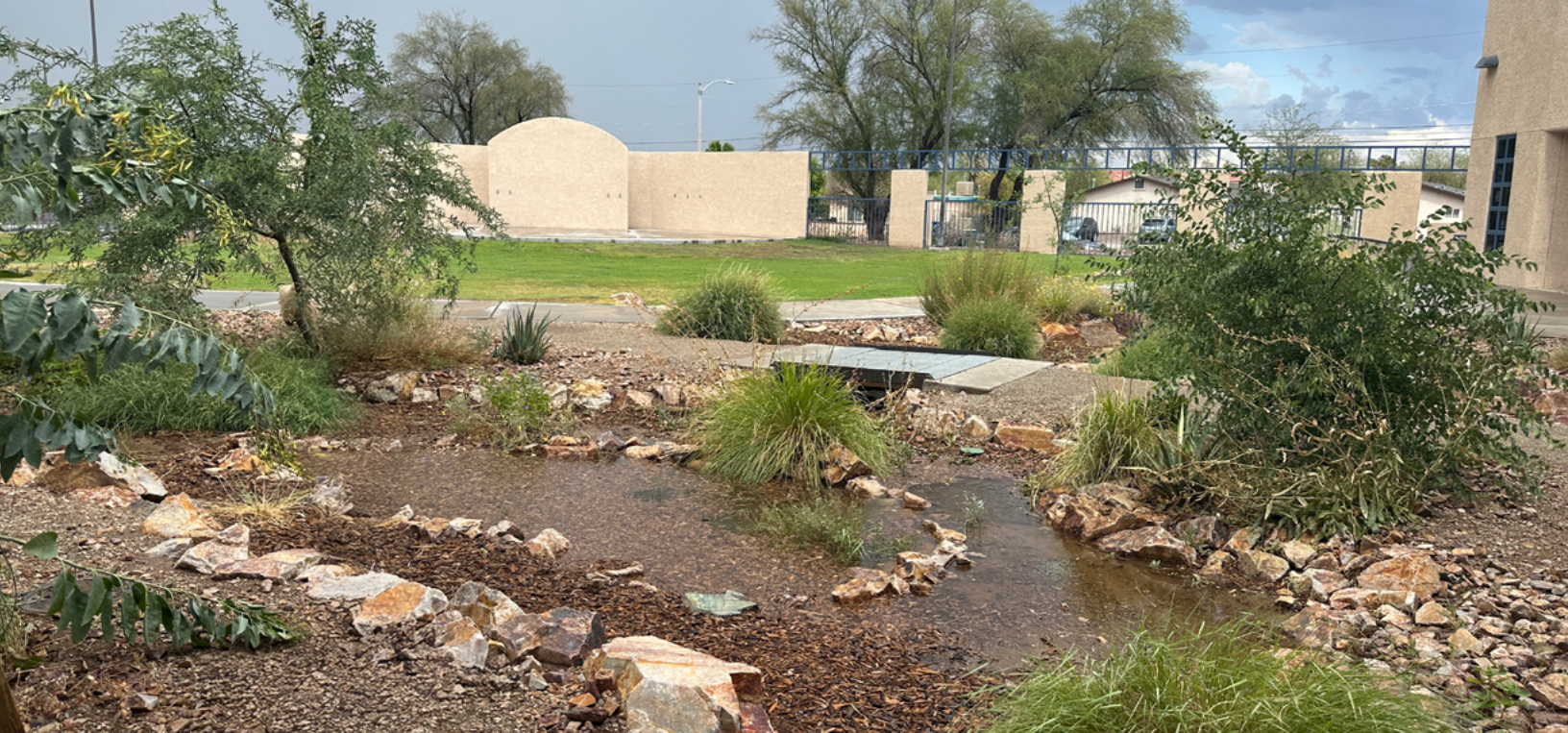
El Rio Neighborhood Center GSI landscape retrofit
